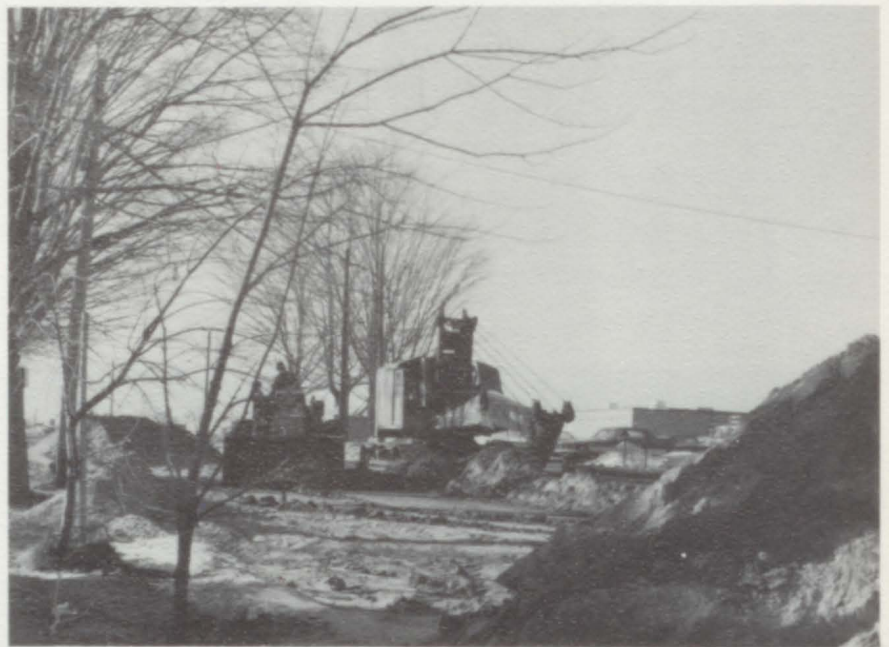
Mayville fights pollution by constructing new sewer system.
